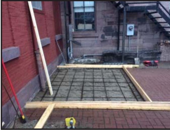
Above, the pad being prepared for the concrete base and below the new unit on the pad.
